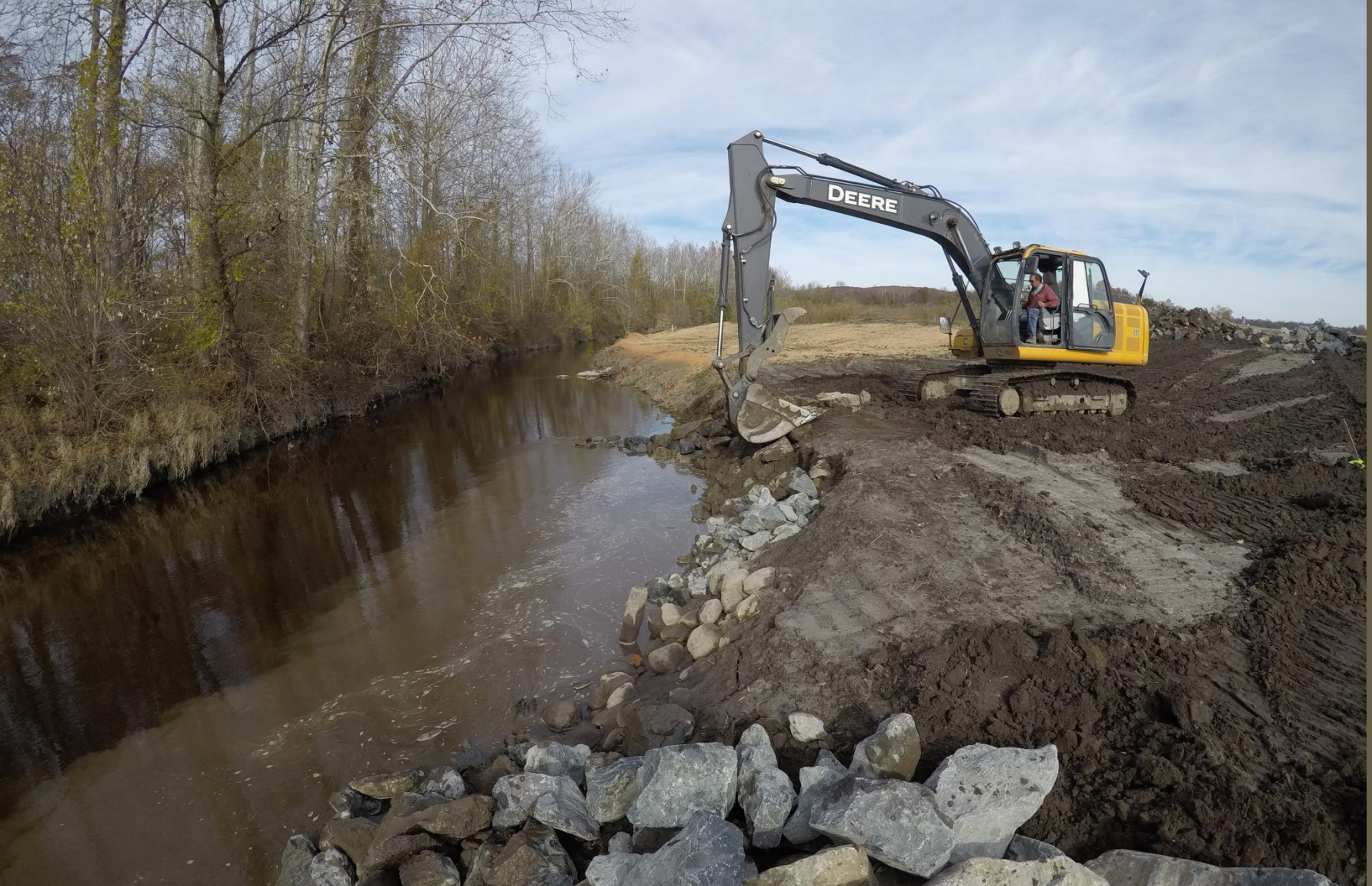
Bank Stabilization- Rock Vanes
