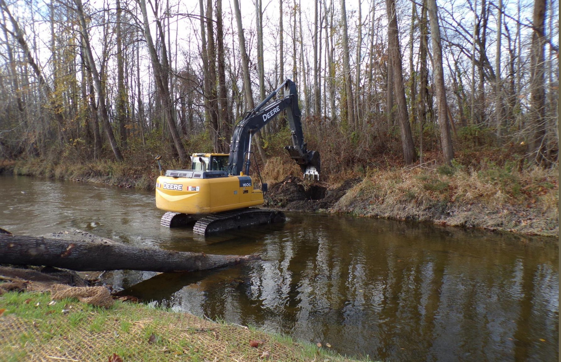
Log Vanes Installed within the Pequest River
