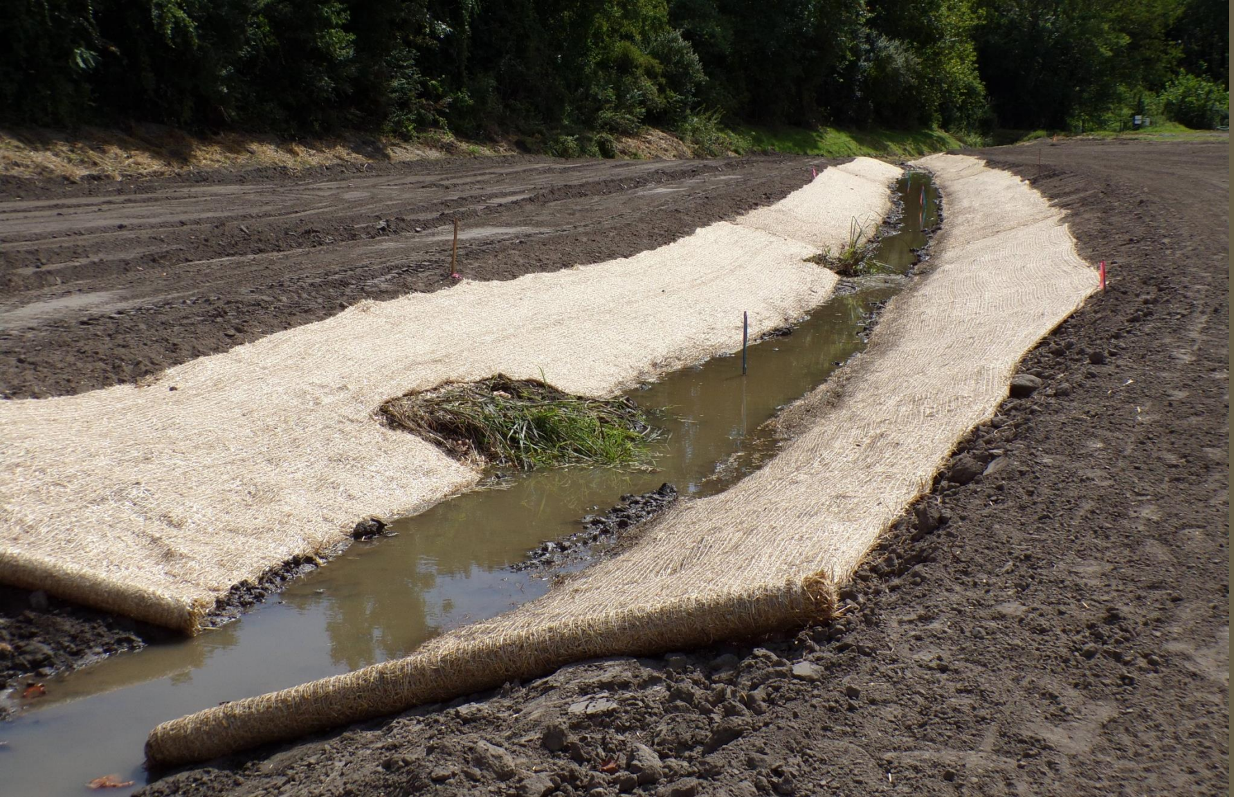
Stabilized Stream Realignment with Plant Salvage
