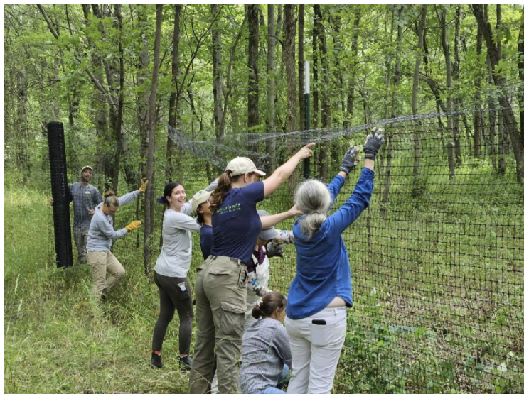
Large plastic fencing installation with our volunteers
